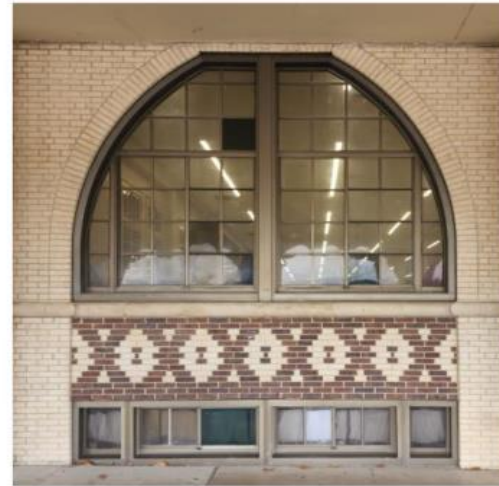
EXISTING CAFETERIA WINDOW
